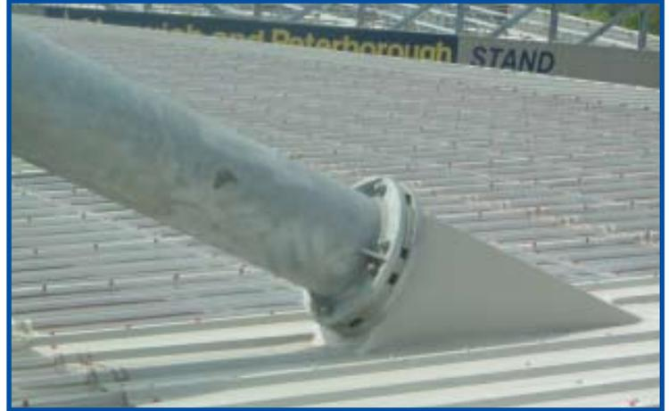
We have successfully completed the weathering of a large number of stadiums where structural columns, supports, ties, struts, cleats etc penetrate various cladding types including composite, single skin, in plane grp rooflight areas, both roof and vertical cladding.
