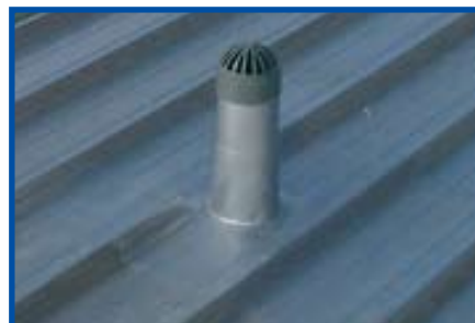
SVP fitted & weathering completed by J&W
